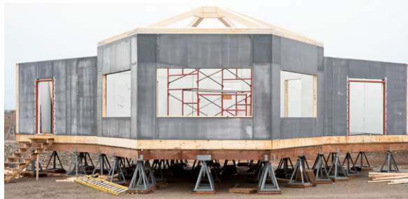
Top: Kuugalak's Elder design committee overseeing the unloading of construction materials. Bottom: The Kuugalak workshop under construction. Photo by Margaret Thompson Photography
